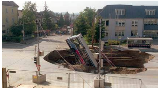
Fig. 10. Collapse of tunnel face Munich underground in September 1994
