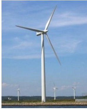
Fig. 2. A typical medium-sized wind turbine.
