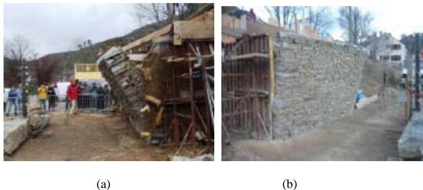
Fig. 3. DSRW tested by Colas et al. (2010b) (a) Failure of a “rural” wall (b) Failure of a “engineered” wall
